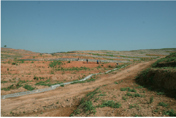
1. Piaoshan section II (view from SE to NW)
